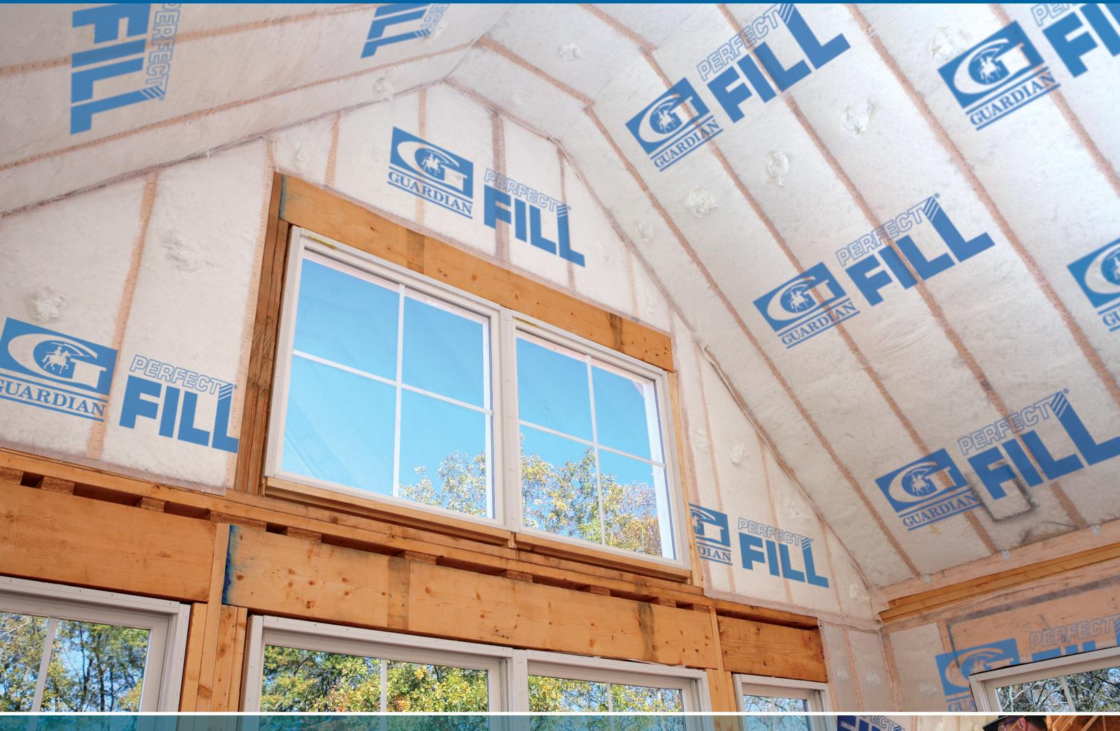
LOOSE-FILL FIBERGLASS INSULATION NETTING SYSTEM
