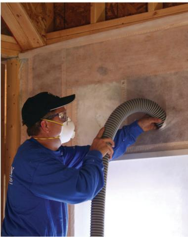
Because of its installed density, Perfect Fill reduces the potential for air infiltration by completely filling small and odd-shaped cavities.
