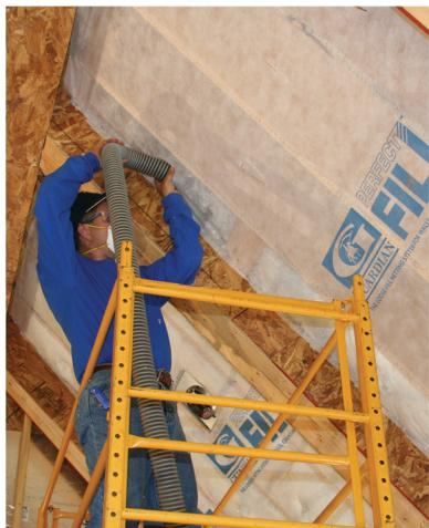
Perfect Fill is the ideal product to properly and effectively insulate vaulted ceilings and sloped roofs.
