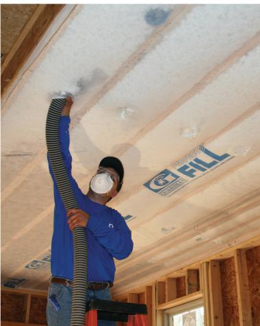
Use Perfect Fill in floors and interior walls to control undesirable noise transfer within the home.
